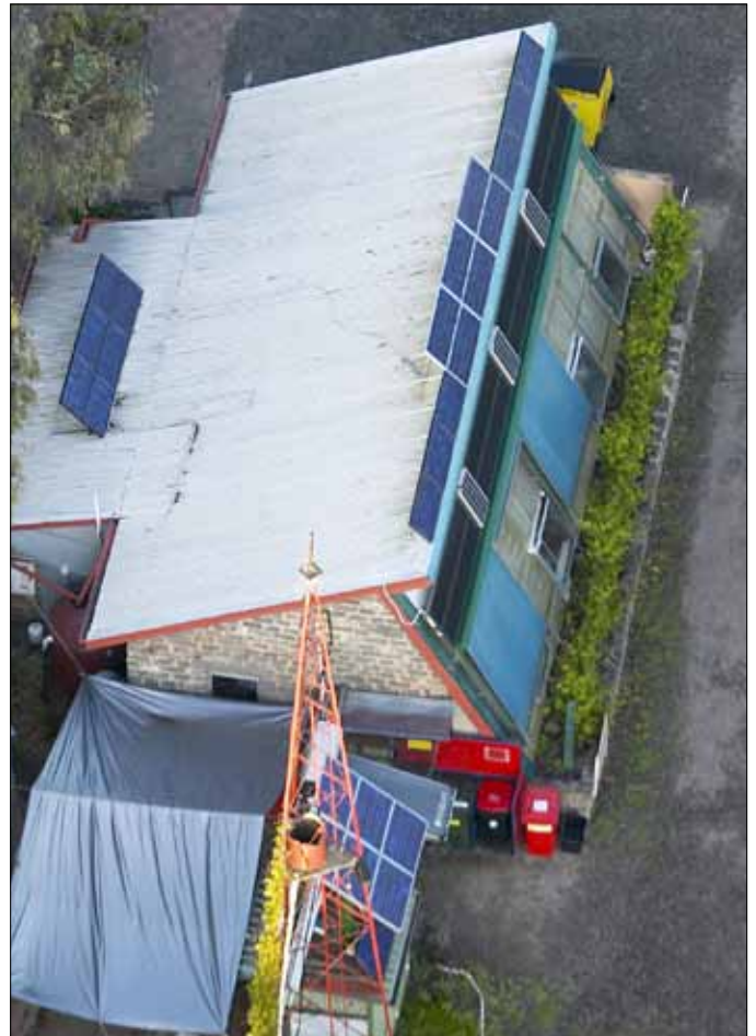
ATA's Solar Workshop at the CERES Environmental Park, Brunswick Victoria, produces solar power that is fed back into the mains electricity grid.
