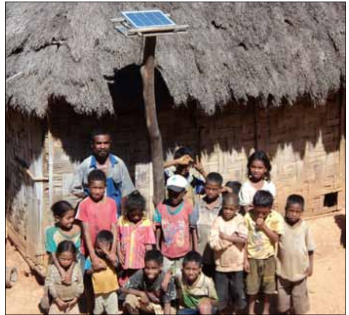
Almost 200 households accessed electricity under the ATA International Project's Village Lighting Scheme.
