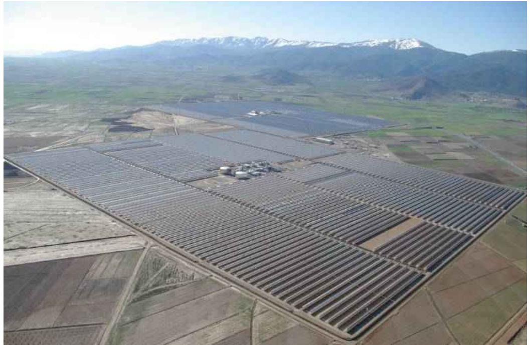
Solar Thermal with Storage
